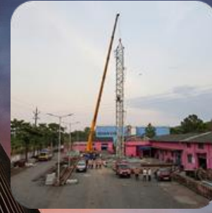
Erection and Commissioning
